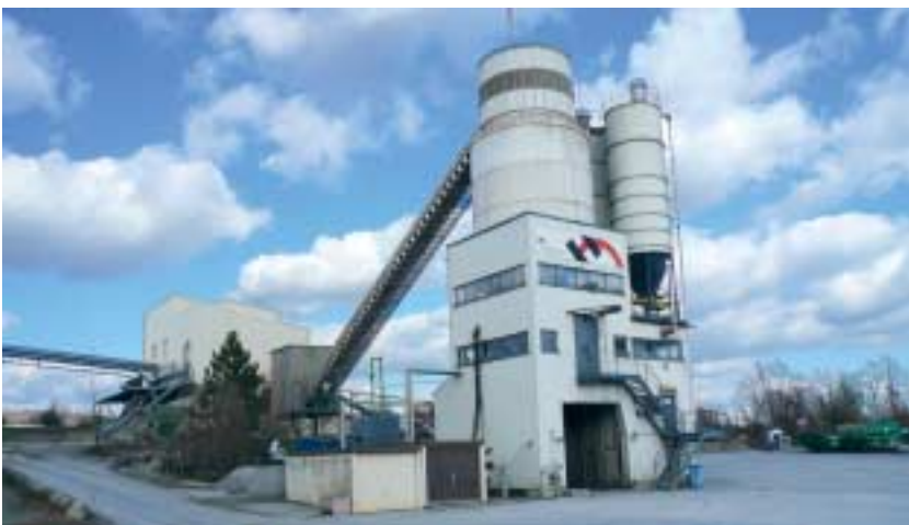
Fig. 1 Concrete plant of Holcim Kies- und Beton AG in Diessenhofen/Switzerland.
