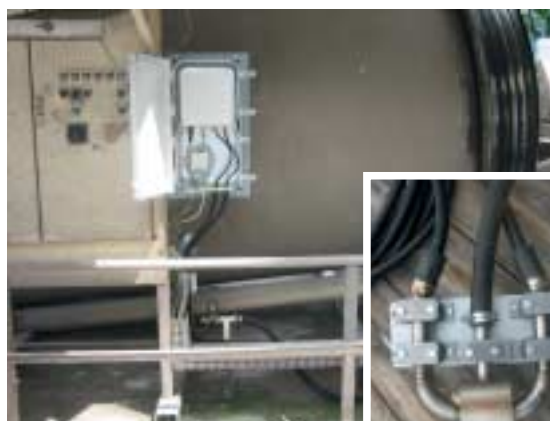
Fig. 3 Measuring electronics mounted in a protection case.
